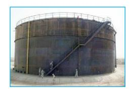
Buried tanks and bunker tanks (partially buried) must have coating or cathodic protection and regular testing of such systems. The bottom of the ASTs may be subject to extensive corrosion, which may not be evident during visual inspections. Corrosion protection can be provided by dielectric coatings and carefully engineered cathodic protection. Some facilities have installed double-bottom tanks to reduce the corrosion factor.
